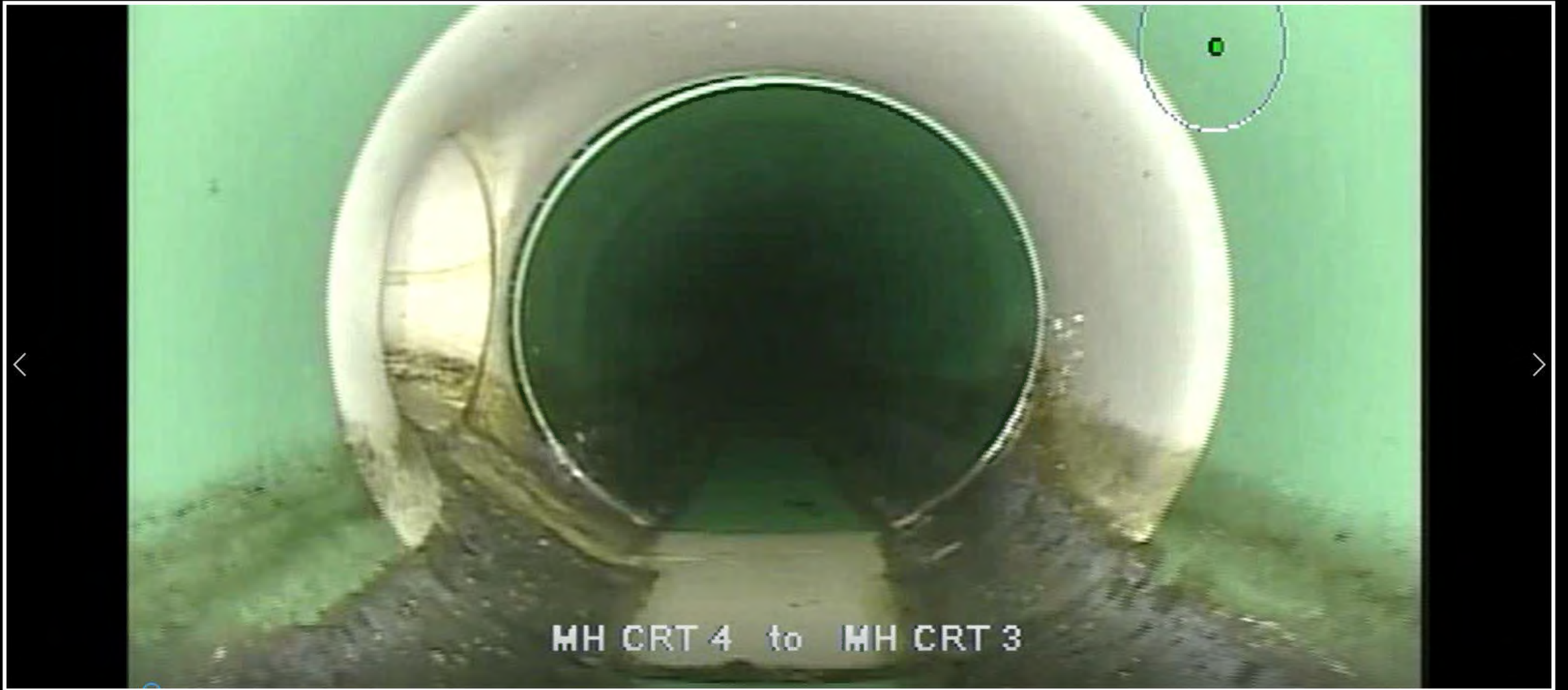
Correct Wye Install
