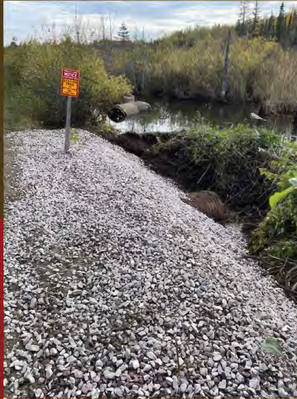
Culvert and trail repair, Tilden
