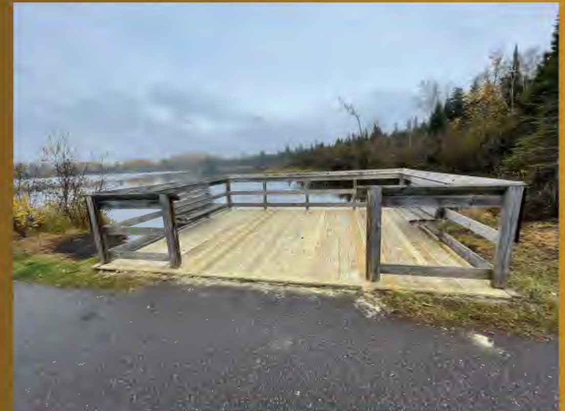
Redecked Section 16 Fishing Dock and fixed split rail fence in Ishpeming
