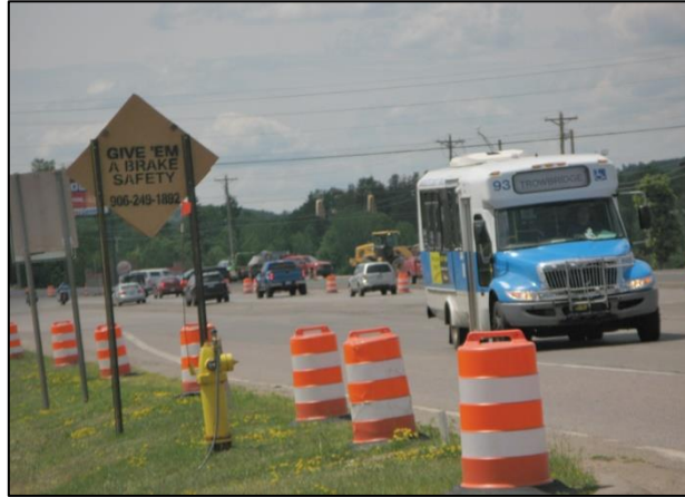
US 41 South road construction
